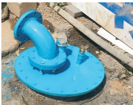
图 8 井口安装 Fig.8 Wellhead installation
