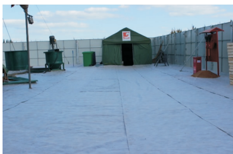
图 8 铺设的环保土工布 Fig.8 Environmental geotextiles
