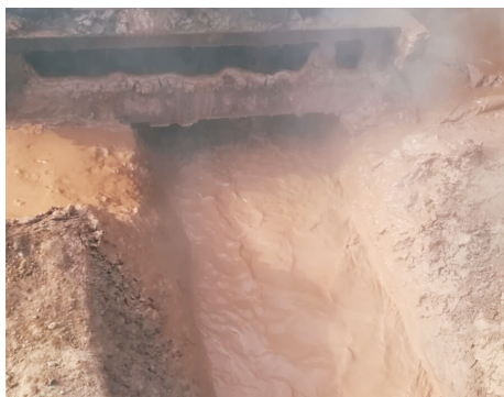
图 4 性能稳定的钻井液 Fig.4 Drilling fluid with stable properties
