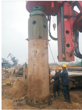
图 3 外护筒与旋挖钻机连接 Fig.3 Connection of outer casing and rotary drilling rig
