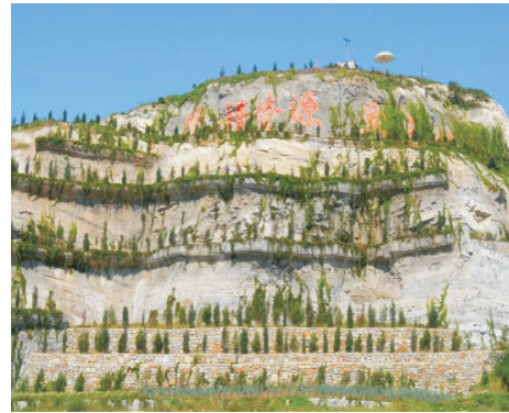
图9 边坡治理后 Fig.9 Slope after treatment
