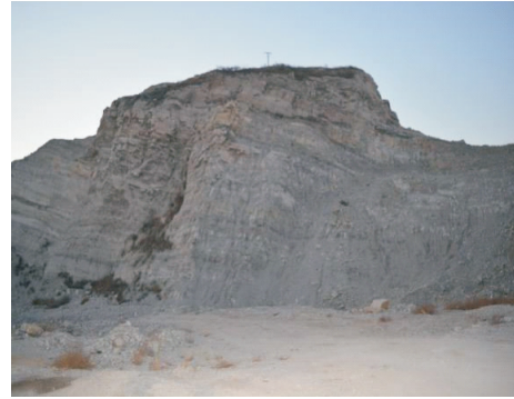
图8 边坡治理前 Fig.8 Slope before treatment
