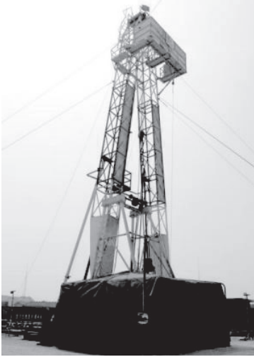
图 1 ZK88-19 钻孔施工现场 Fig.1 ZK88-19 drilling site
