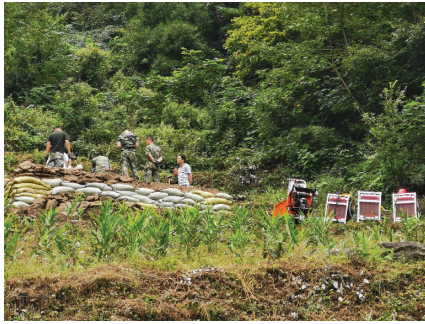
(a) 钻探场地修筑
