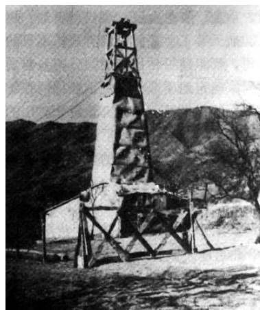
图 1 1949 年 7 月地质部门解放后第一台钻塔耸立在北京门头沟矿 Fig.1 The first derrick of geology industry of the New China erected in Beijing Mentougou Mine after liberation in July 1949
