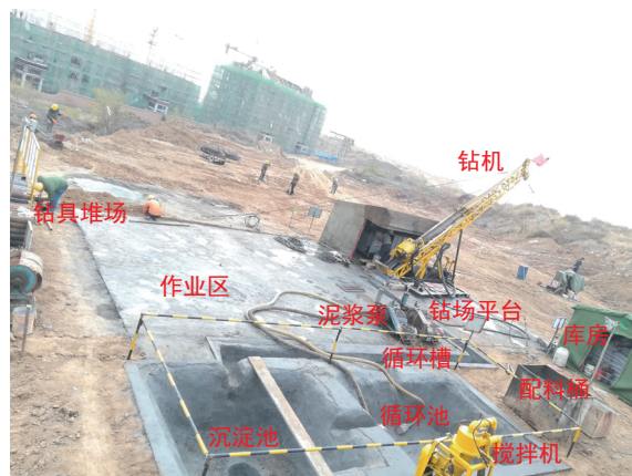
图3 处理后的钻场及冲洗液循环系统 Fig.3 Post-treatment drilling site and fluid circulation system
