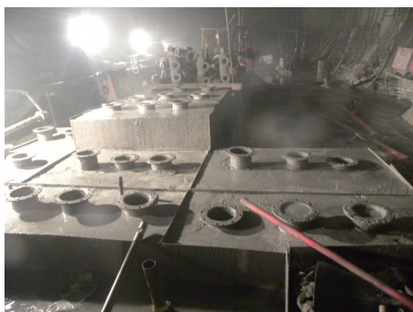
图 6 注浆孔口管预埋及砼浇筑后的沉箱效果 Fig.6 Caisson with the pre-embedded grouting pipe and cast concrete
