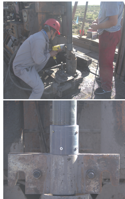
图6 PVC-U套管下管方式及连接固定 Fig.6 Running-in-hole mode and connection of PVC-U casing
