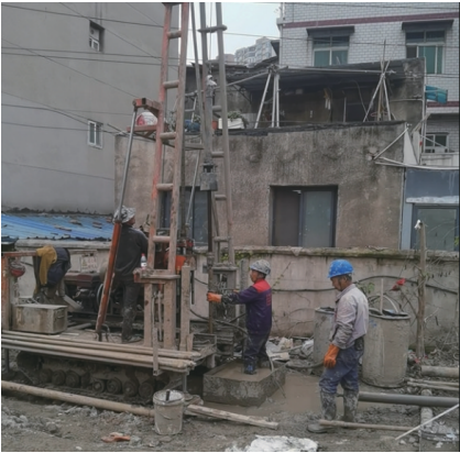
图2 钻孔取样现场作业情况 Fig.2 On-site sampling operation
