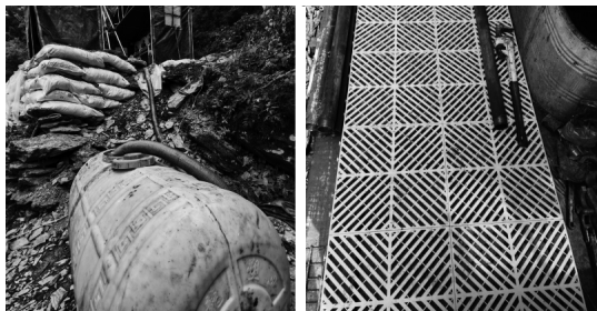
(a) 冲洗液沉淀 (b) 机台内铺设防滑地格栅
